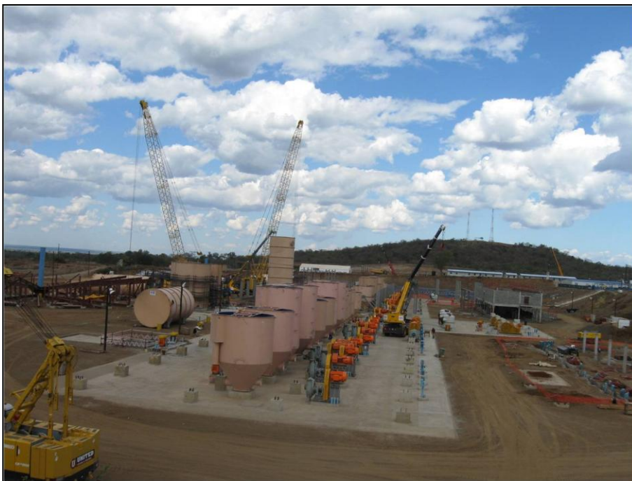
Figure 19: Processing Plant under Construction – June 2010
