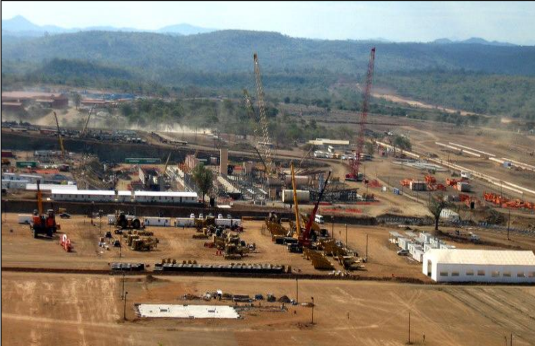
Figure 15: Construction of CHPP and Mine Infrastructure Underway
